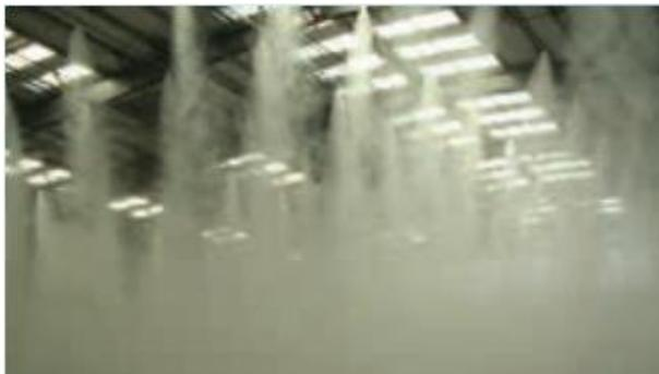
*Fig. 3 Example of high-pressure object protection system (Source: Author)*
